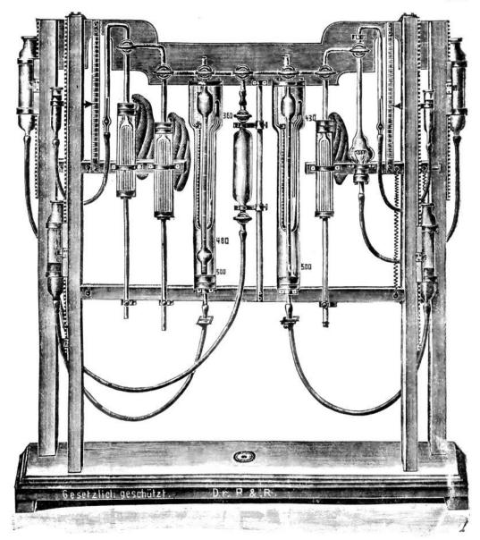
the simplest, quickest and most exact manner according to Sections 71 and 72 of the general mining police order, January 18, 1900, of the Royal Head Mining Office, Breslau. The apparatus serves further for the determination of methane in the high nitrogenous gases which are found in mine inflammatory gases. It is also quick and accurate for determining their content of carbon monoxide. F. SCHREIBER.
